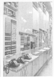
No. 1 Crossbar switch, developed late 1930s
