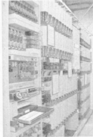
Step-by-step switch, typical of the type that brought dial service to many smaller communities
