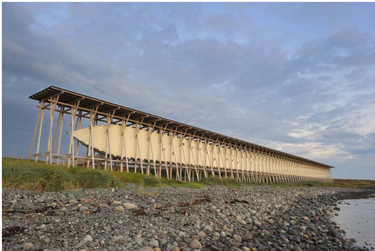
The elongated wooden construction designed by Peter Zumthor refers to a Norwegian tradition: the racks for drying codfish. © Photo: Jarle Wæhler / Statens vegvesen
