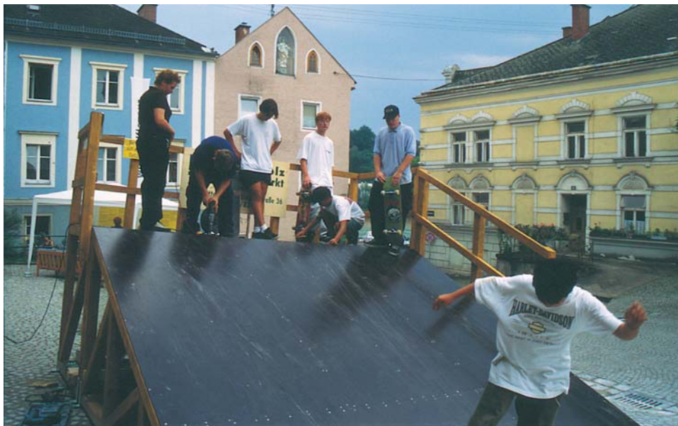
Ottensheim skater ramp construction
