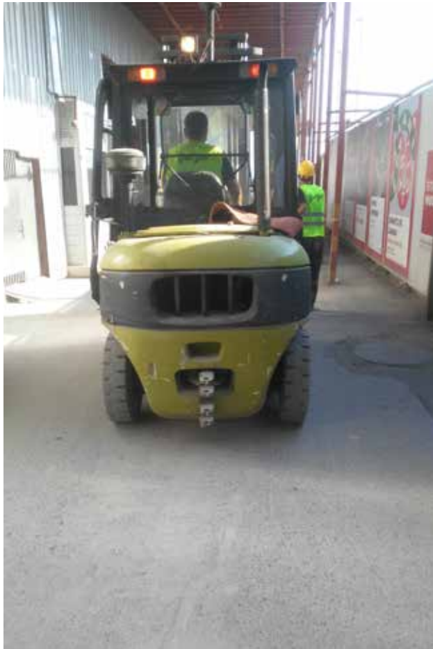
Construction outside of Istanbul Modern, 2017, Photograph by: Amy Bruce
