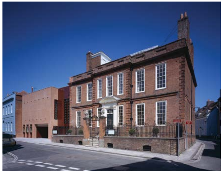
Fig. 2: Pallant House Gallery exterior. © Peter Durant.
