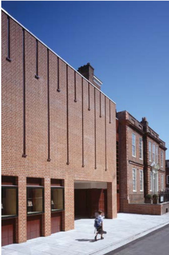
Fig. 1: Pallant House Gallery exterior. © Peter Durant.
