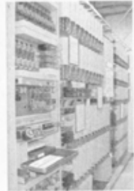
Step-by-step switch, typical of the type that brought dial service to many smaller communities
